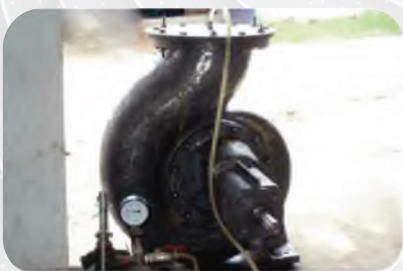
HYDRO LEAK TESTING
